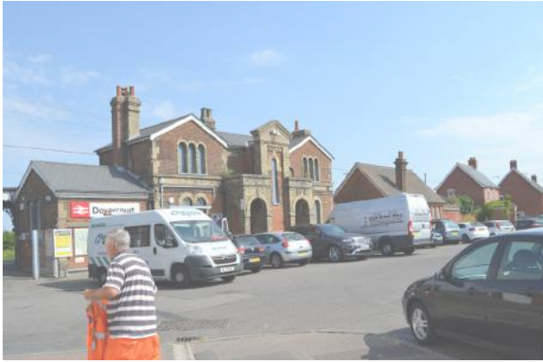
Existing view of Dovercourt Station
