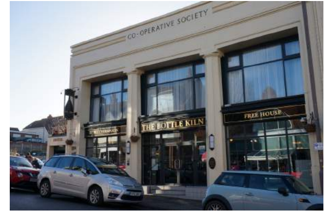
The Bottle Kiln Wetherspoon Pub in the former Co-op Store has restored a previously dilapidated buildings and turned it into a new eating-out destination
