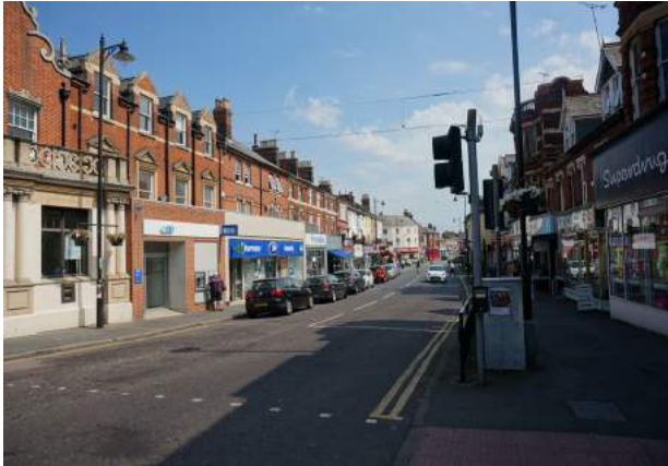
Fine grain parade of shops characterise the High Street in the centre, albeit the quality of shop fronts is frequently poor and detracts from the character of the street
